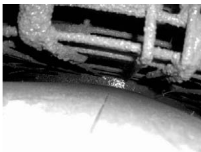
Fig. 8a. During the concreting.
