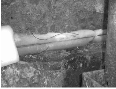
Fig. 4. Preparing works and using of Lamposilex, as a water stopping material.
