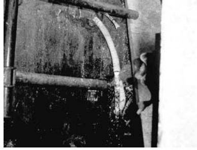
Fig. 4. Preparing works and using of Lamposilex, as a water stopping material.
