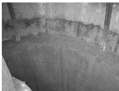
Fig. 8b. After concreting.
