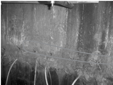
Fig. 5. Using the Resfoam 1KM for the injection with the packers.
