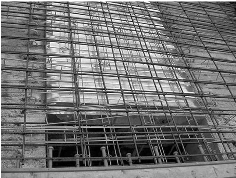
Fig. 5. Longitudinal and transverse reinforcements are CFRP rebars in the two mile creek bridge.
