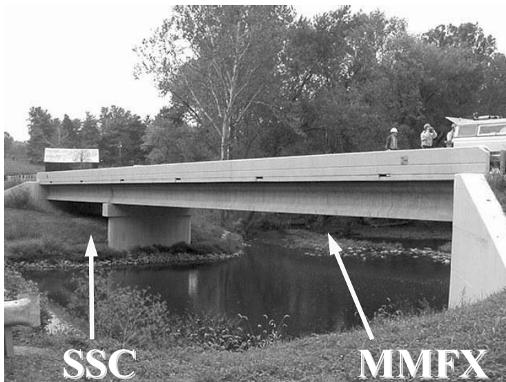
Fig. 8. SSC and MMFX bars were used in the bridge deck of the CR 5218 Bridge in Scott County, Kentucky, USA.
