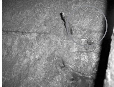
Fig. 5. Using the Resfoam 1KM for the injection with the packers.
