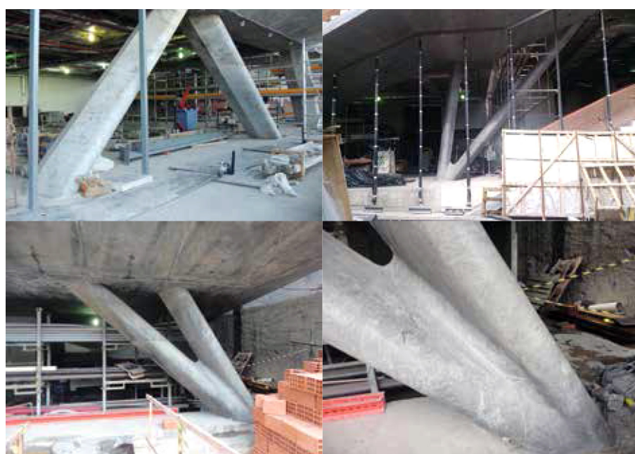
Fig. 6: Actual inclined columns in the building exhibit the high-quality finishes required of the exposed structural and architectural elements
