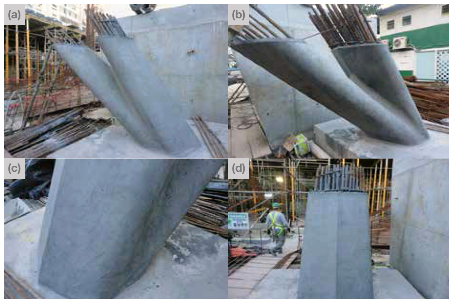
Fig. 5: Mockup finishes: (a) sides; (b) sides and lower region at joint; (c) detail at base and joint; and (d) overview of upper inclined region
