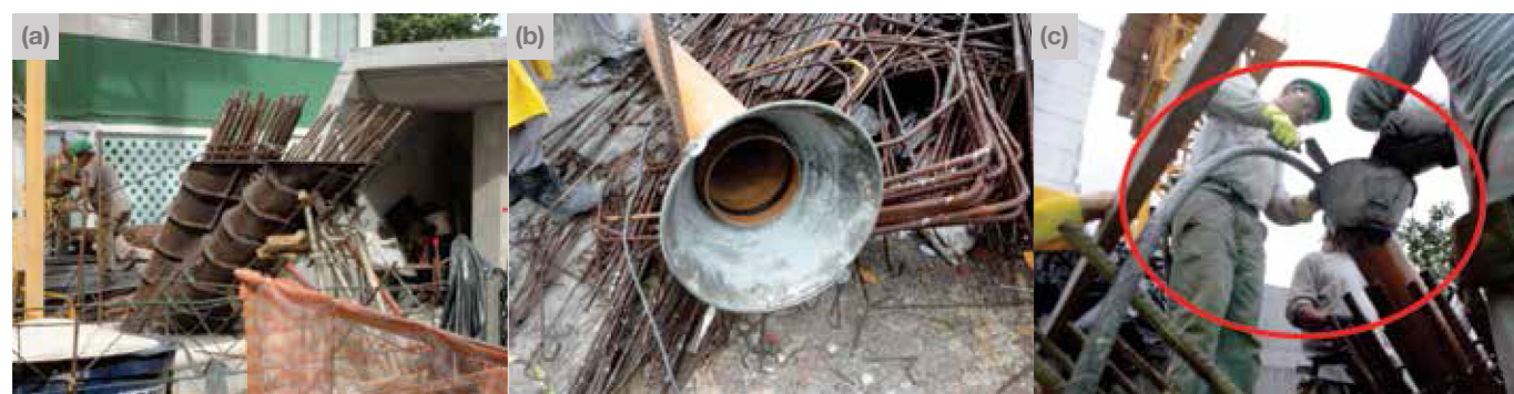
Fig. 4: Casting the inclined column mockup helped in the evaluation of various factors: (a) metal forms and inclined reinforcement projected from a previously cast base joint; (b) a drop tube was used to deliver concrete from the concrete bucket to the base of the column form; and (c) a bottomless pail acted as a funnel and reservoir for concrete, allowing a vibrator to be inserted into the drop tube without overflow
