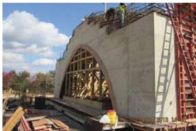
Fig. 8: The mosque structure included a platform for the main dome supported on four arched beams. The arched beams were formed using a combination of shored structural laminated timber to form the arch and PERI TRIO panel formwork to form the sides
