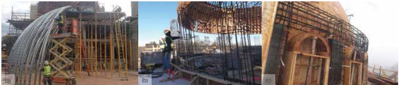
Fig. 9: The primary dome on the mosque was too large to be formed using EPS foam, so custom formwork was fabricated from crimped cold-formed steel shapes and plywood sheathing: (a) the Radius Track cold-formed shapes were assembled at the ground level; (b) the partially completed assembly was installed using a tower crane; and (c) the remainder of the dome formwork sheathing was fastened to the framing and the window formwork was installed
