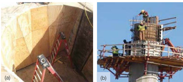
Fig. 11: The minarets comprise rectangular bases and polygonal towers: (a) the transition between base and tower was formed using dimension lumber and plywood sheathing; and (b) the tower was formed using a hybrid system comprising MevaLite wall formwork, dimension lumber, and plywood sheathing lifted into place using the site's tower crane
