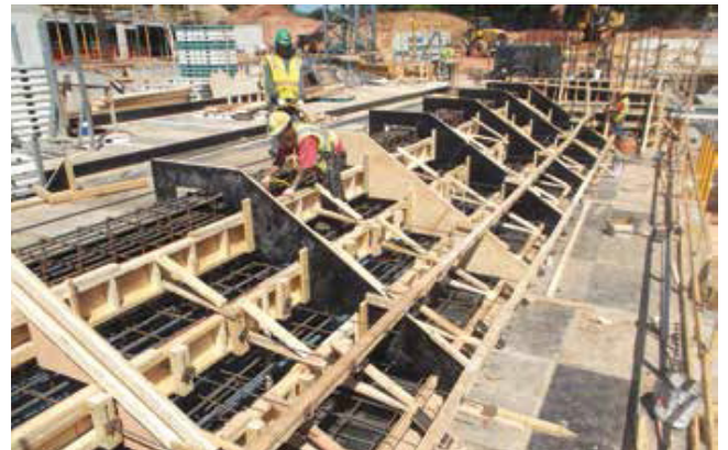
Fig. 12: Seating areas in the Turkish bath were formed using dimension lumber and plywood sheathing
