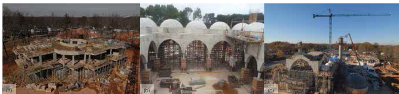
Fig. 6: Multiple shoring and decking solutions were used for construction of the project: (a) elevated floors in the Turkish bath were formed using PERI MULTIPROP shoring, formwork girders, SKYDECK panel slab formwork supplied by PERI Formwork Systems, Inc., along with HICO beams provided by Form Service, Inc. (photo courtesy of Mostafa Fahimi, EyeConstruction, Inc.); (b) formwork for the small domes surrounding the mosque courtyard were supported on Harsco 20K steel shoring (photo courtesy of Facchina Construction Company, Inc.); and (c) support for the main dome arch formwork and the work platform below the main dome formwork were provided by Harsco GASS aluminum shoring and joists
