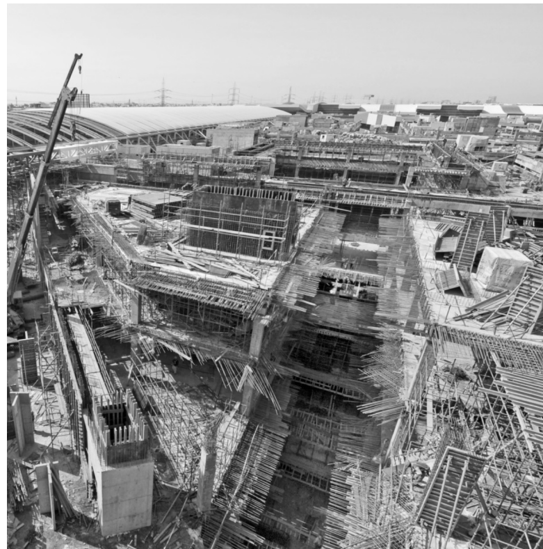
The Avenues, Phase 3, Soku extension and West Village construction
