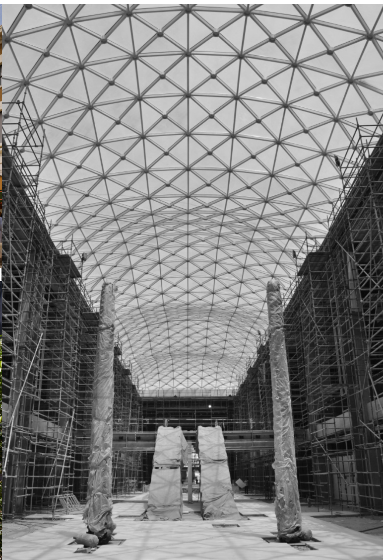
The Avenues, Phase 3, Skylight along Prestige Street
