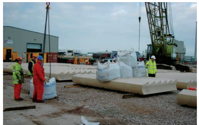
Load testing of the revetment units
