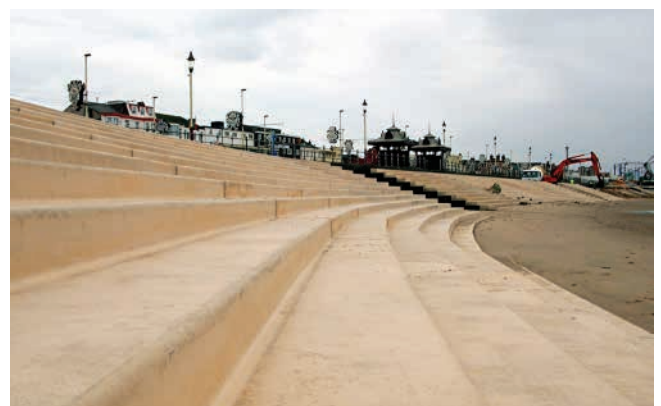
Some of the first revetment units in place
