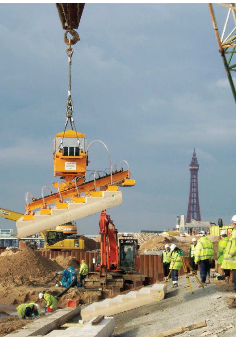
Vacuum machine lowering precast unit
