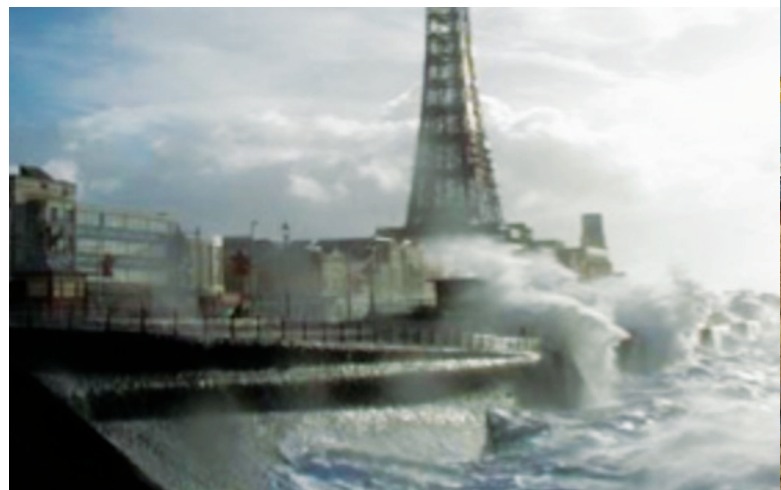
The old sea wall during a major storm
