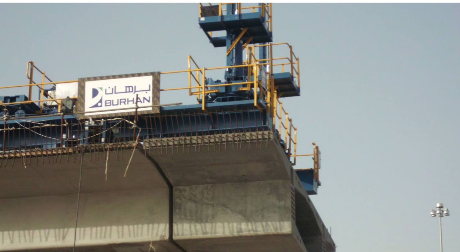
Element in place
