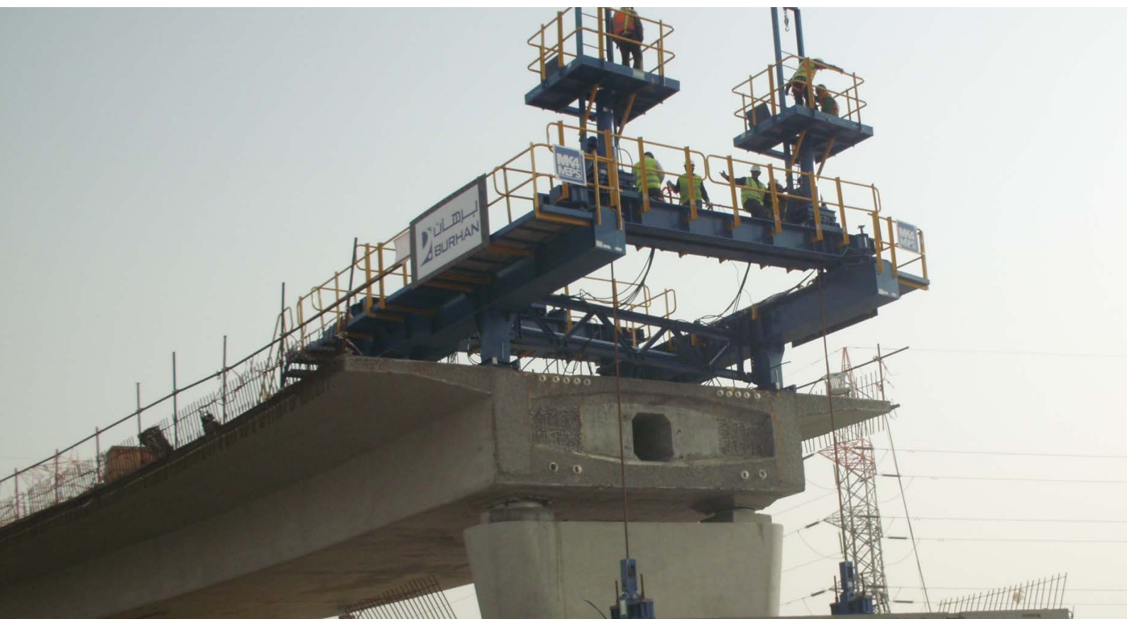
Lifting of first element at column
