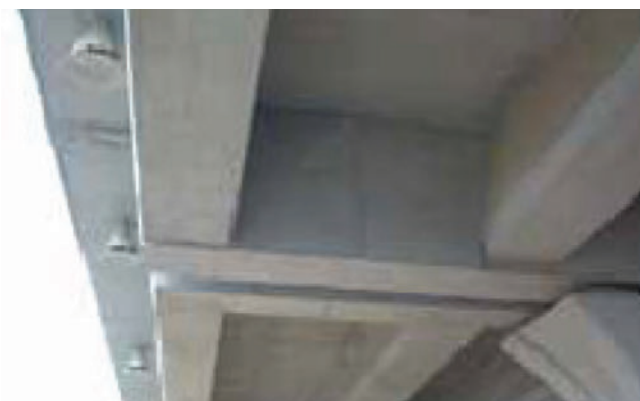
Figure 1a: Photograph of the soffit of a flyover
