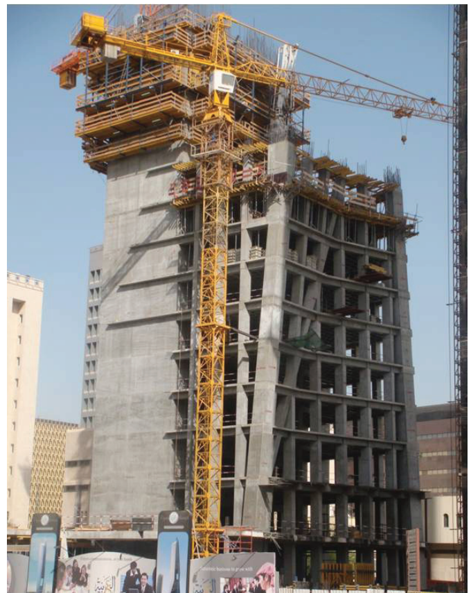
Crystal Tower during construction
