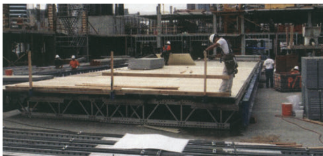
Column-hung flying deck forms being built up on a job site. Trusses span between girders that will be supported by columns
