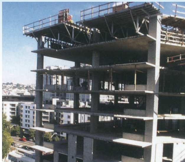
Conventional flying form trusses immediately after flying. Reshores will be installed prior to placing the slab
