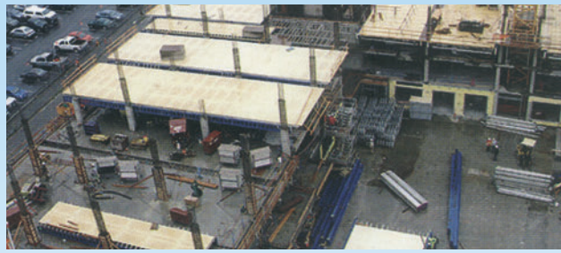
Aligned columns facilitate a clean formwork layout and maximize productivity
