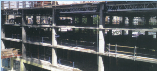
Column-hung flying deck forms prior to placing the slab. All slab loads are carried directly by the columns, resulting in open decks below the forms with no shores or reshores. This allows workers to move about freely
