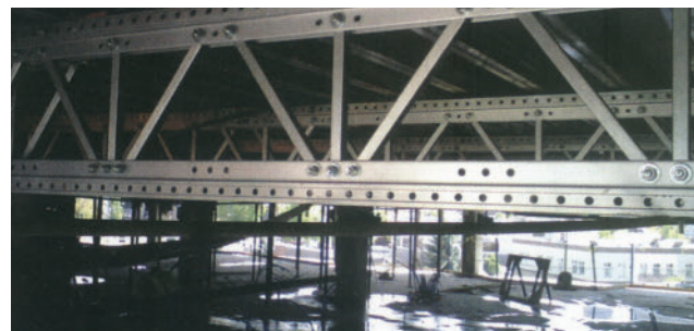
The trusses supporting these flying deck forms are fully adjustable, allowing versatility in span and spacing
