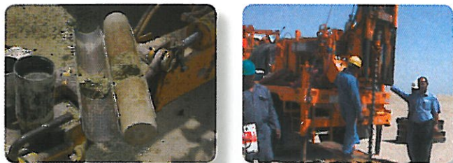
Fig. 3. Subsurface explorations by borehole drilling.
