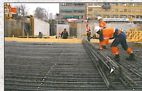
Fig. 3: At the construction site, the prefabricated reinforcement carpets can be laid in less than 80% of the usual time
