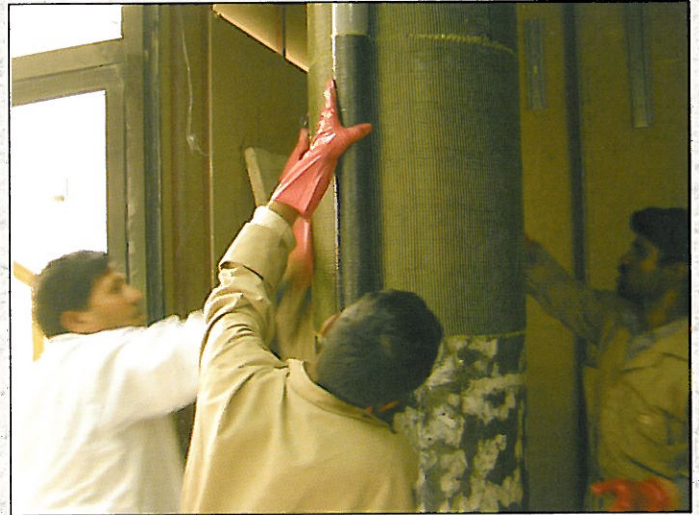
Figure 2 Fitting layers of CFRP.
