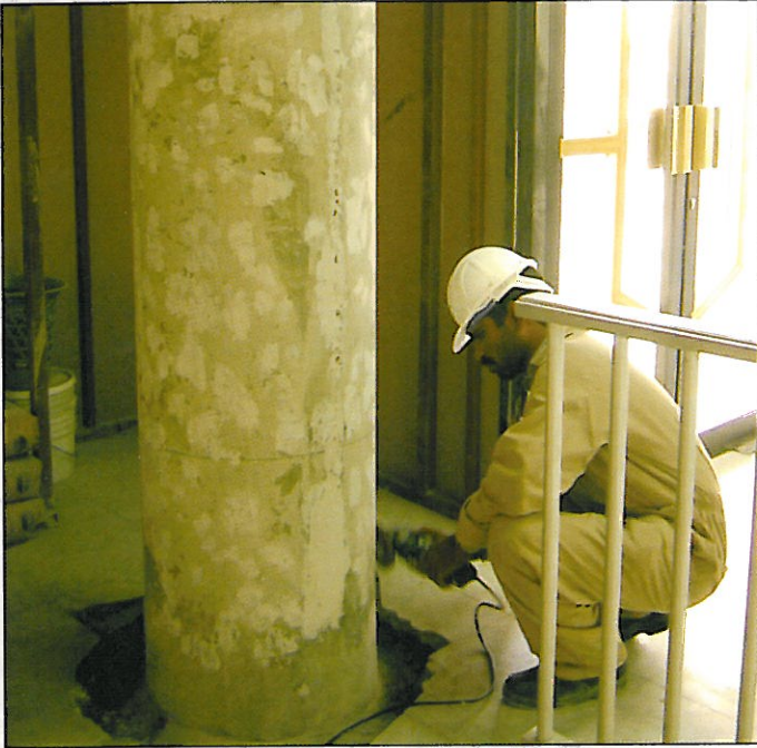
Figure 1 Surface preparation.
