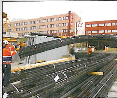
Fig. 1: At the job site, cranes are used to transport the reinforcement elements (carpets) manufactured using bamtec reinforcement technology
