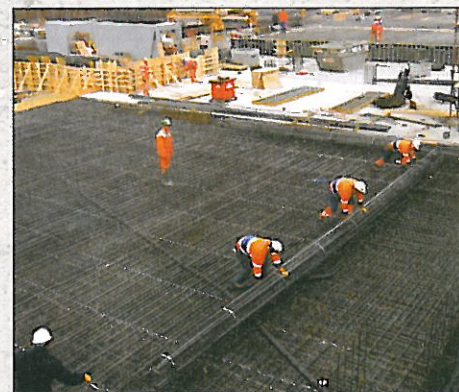
Fig. 2: Installation of a reinforcement element (carpet) manufactured using BAMTEC reinforcement technology
