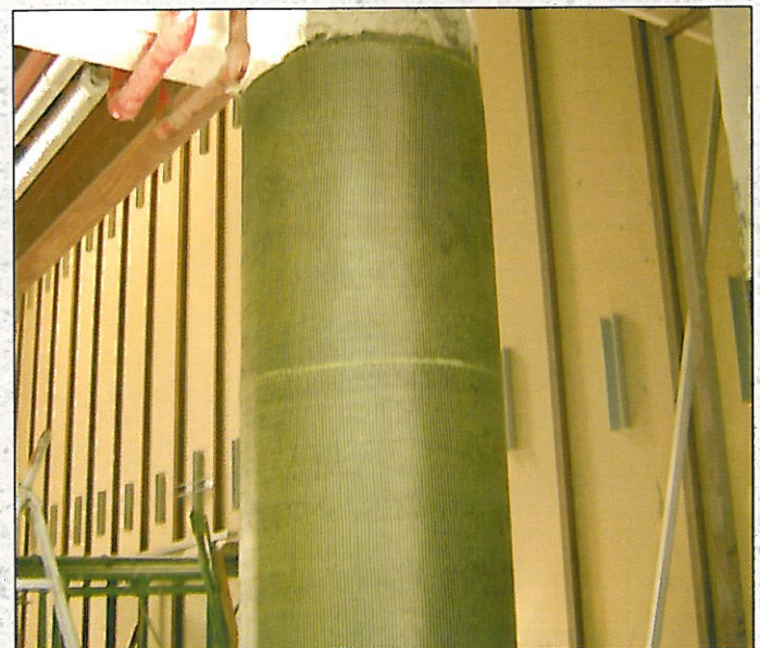
Figure 3 The final shape of CFRP.
