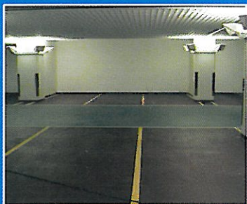
Car Park System
