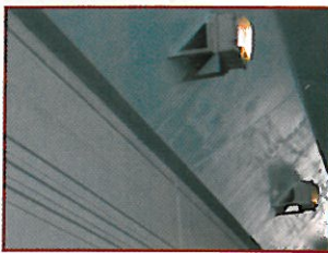
Detail of Completed Bracket
