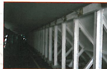
Formwork Ready for Concrete
