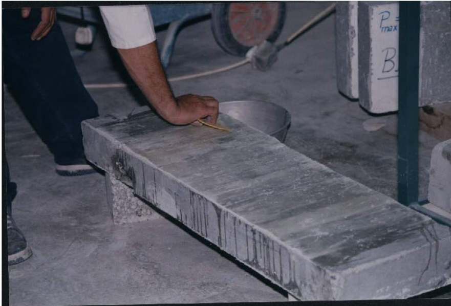
Figure 4: Application of CFRP fabrics
